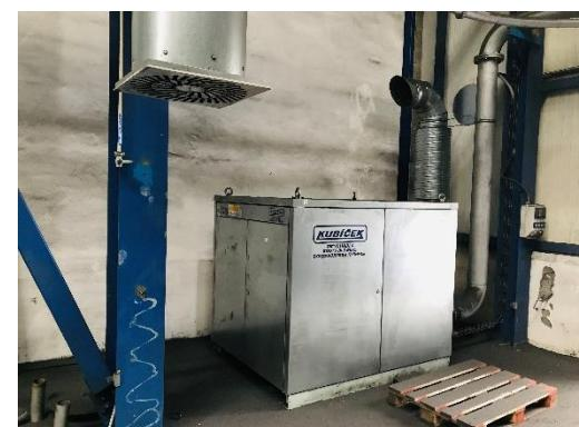
Inlet air-conditioning units with heating and recuperation
