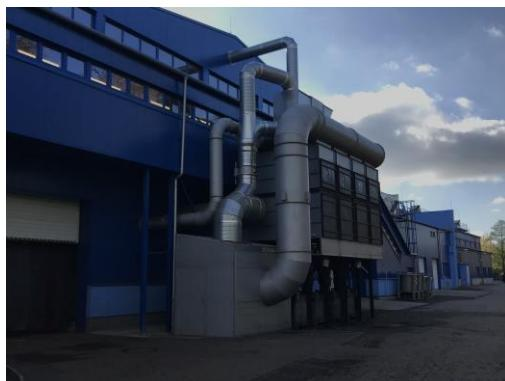
Alignment of the knock-out grid and piping
