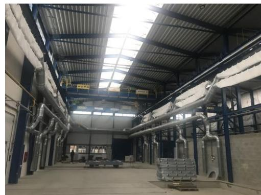
Filtration equipment F 02 for capturing solid pollutant particles from the knock-out grid
