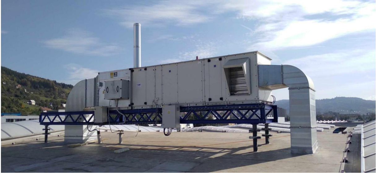
Industry air handling unit with a capacity of 15 000 m 3 /h, gas burner.
