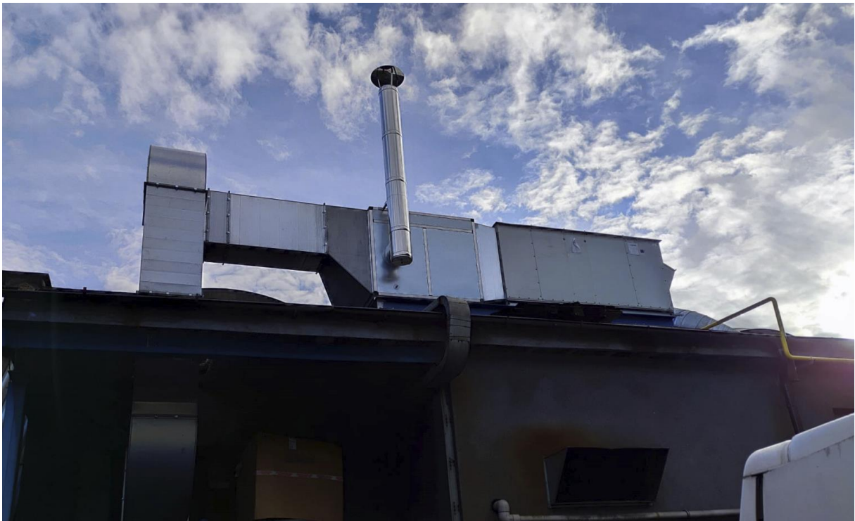
Industry air handling unit with a capacity of 30 000 m 3 /h, gas burner.
