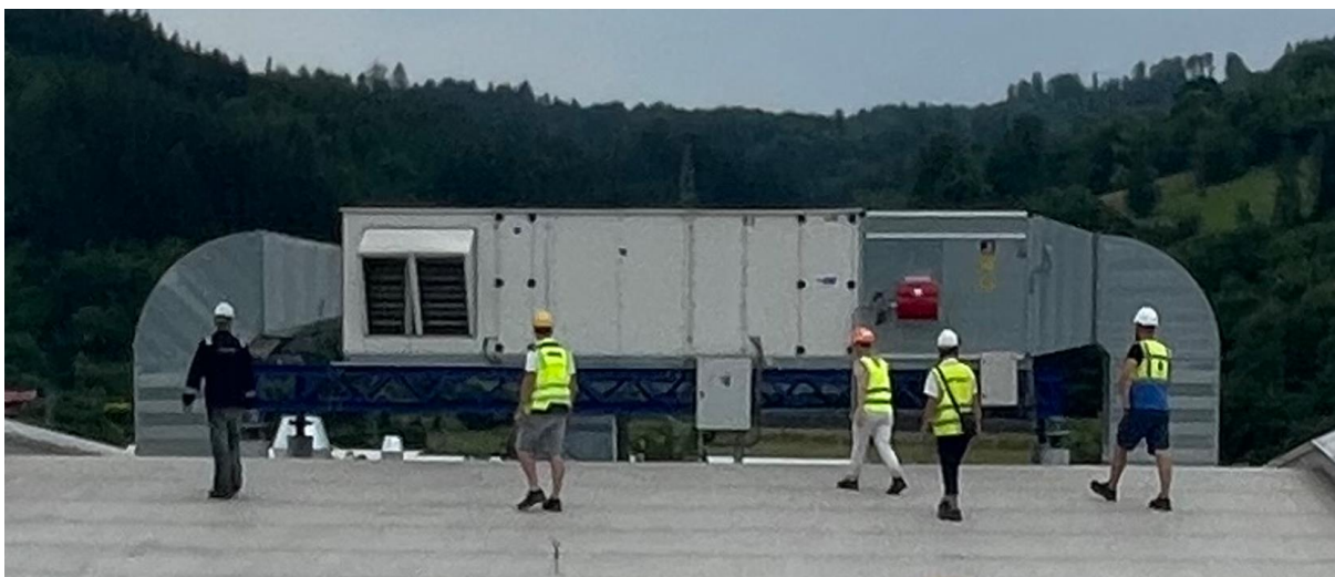
Industry air handling unit unit with a capacity of 24 000 m 3 /h, electric heating.
