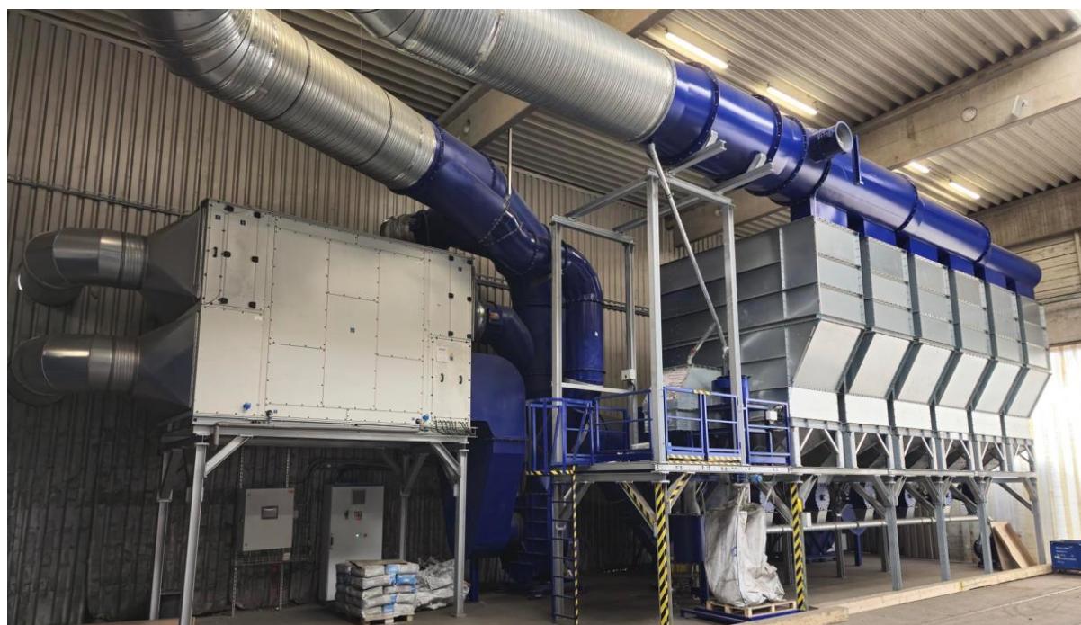
Figure 3 Filtration unit with supply air heat recovery unit
